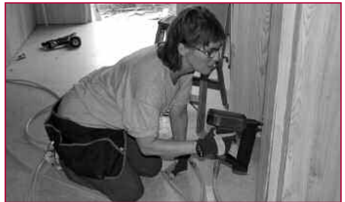
IRT volunteer helps repair home of Hurricane Katrina victims.
